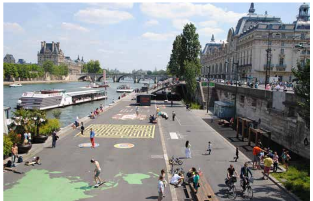
Paris, Left Bank: the stair deck in front of Musée d'Orsay and the space created on the former expressway. Copyright: Paul Lecroart/Institut Paris Region
