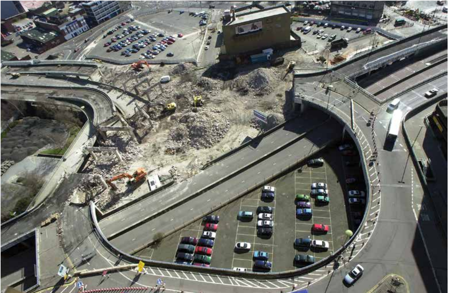
Birmingham: demolition of Masshouse Circus in 1990s. Copyright: BPM Media
