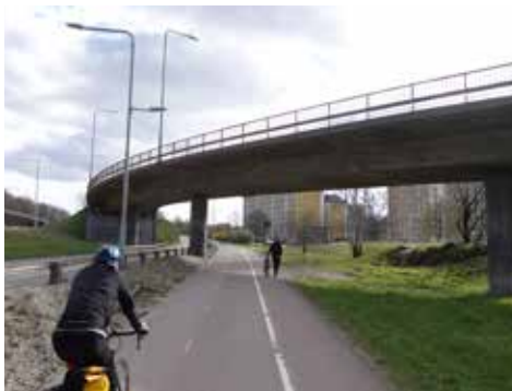
The existing segregated highway
