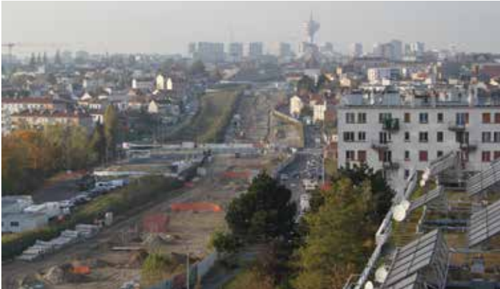
Before: demolition of the A186 highway. Copyright: Paul Lecroart/Institut Paris Region
